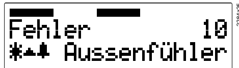
Example of own fault display
